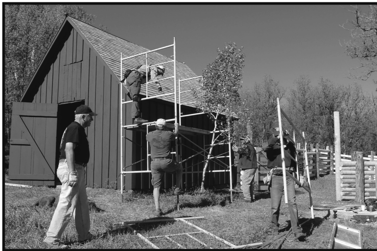
Building Restoration & New Fence
